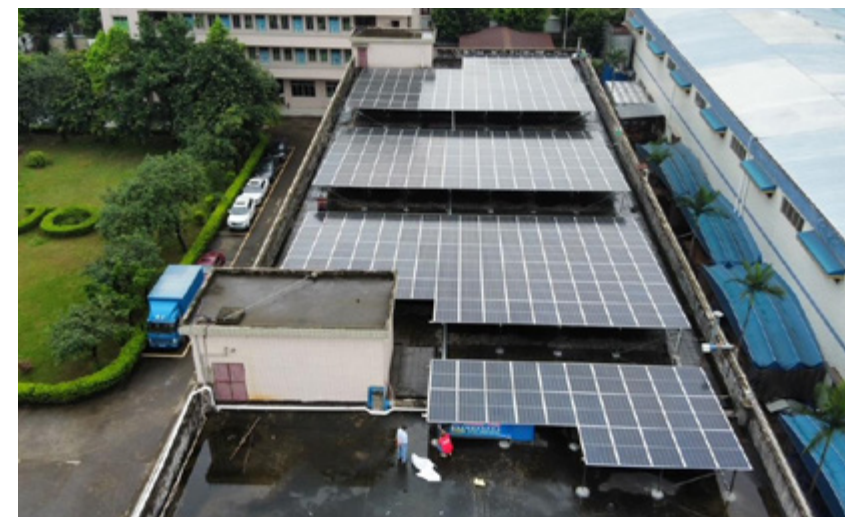
The solar power generation system installed in Foshan site with a power generation capacity of 209,829 KWH in 2023.
